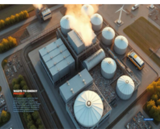
Solid waste management and waste-to-energy project
